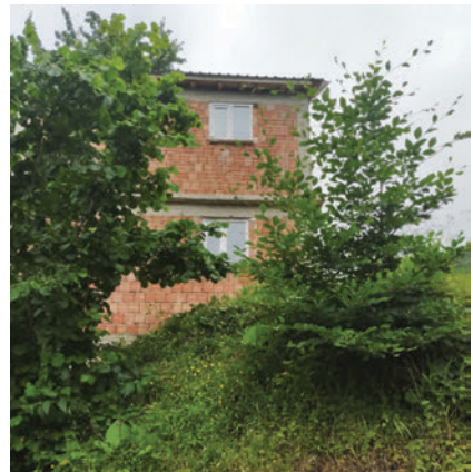
After the renovation
